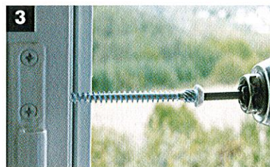
3 Vissage direct auto-perceuse
